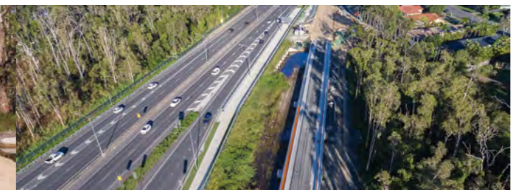
BIGGERA CREEK BRIDGE LOOKING WEST ALONG THE SMITH STREET MOTORWAY.
