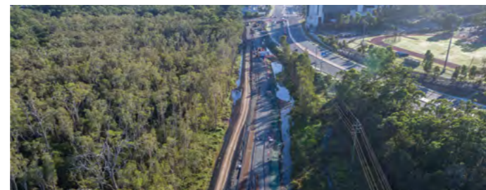
OLSEN AVENUE LOOKING NORTH TOWARDS GRIFFITH UNIVERSITY AND THE GOLD COAST UNIVERSITY HOSPITAL.
