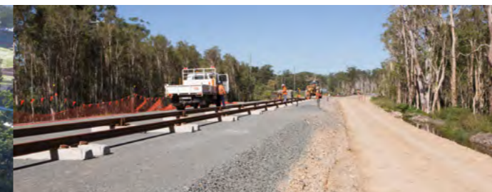
OLSEN AVENUE LOOKING SOUTH TOWARDS THE SMITH STREET MOTORWAY.
